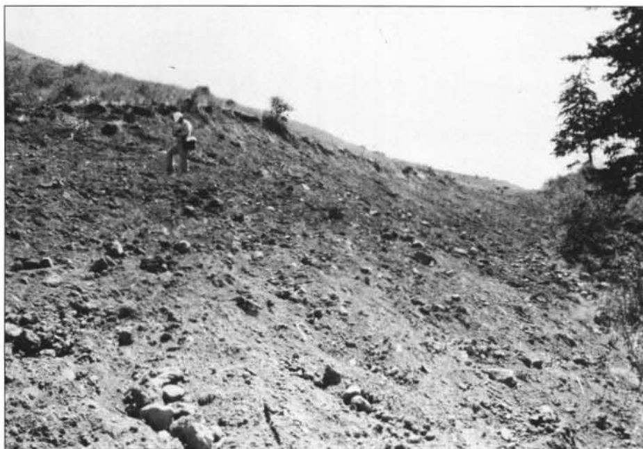
Figure 1. Road reclamation in progress at the Cannon Mine, Washington. These slopes have been reshaped to match the local natural slopes. Seeding is done at first planting season after reshaping to minimize erosion.
