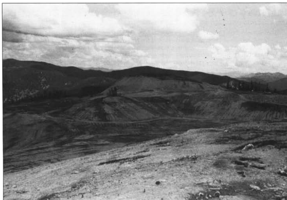
Figure 4. Reclaimed Sunnyside pit at Coeur d'Alene Thunder Mountain Mine. Pit walls have been worked into sinuous contours and rolling topography. Newly planted vegetation has endured two years of drought. Lodgepole pines, which were severely stressed, show excellent recovery and growth after heavy winter snows and a wet summer. Grasses, although still sparse, continue to spread and provide seeds.
