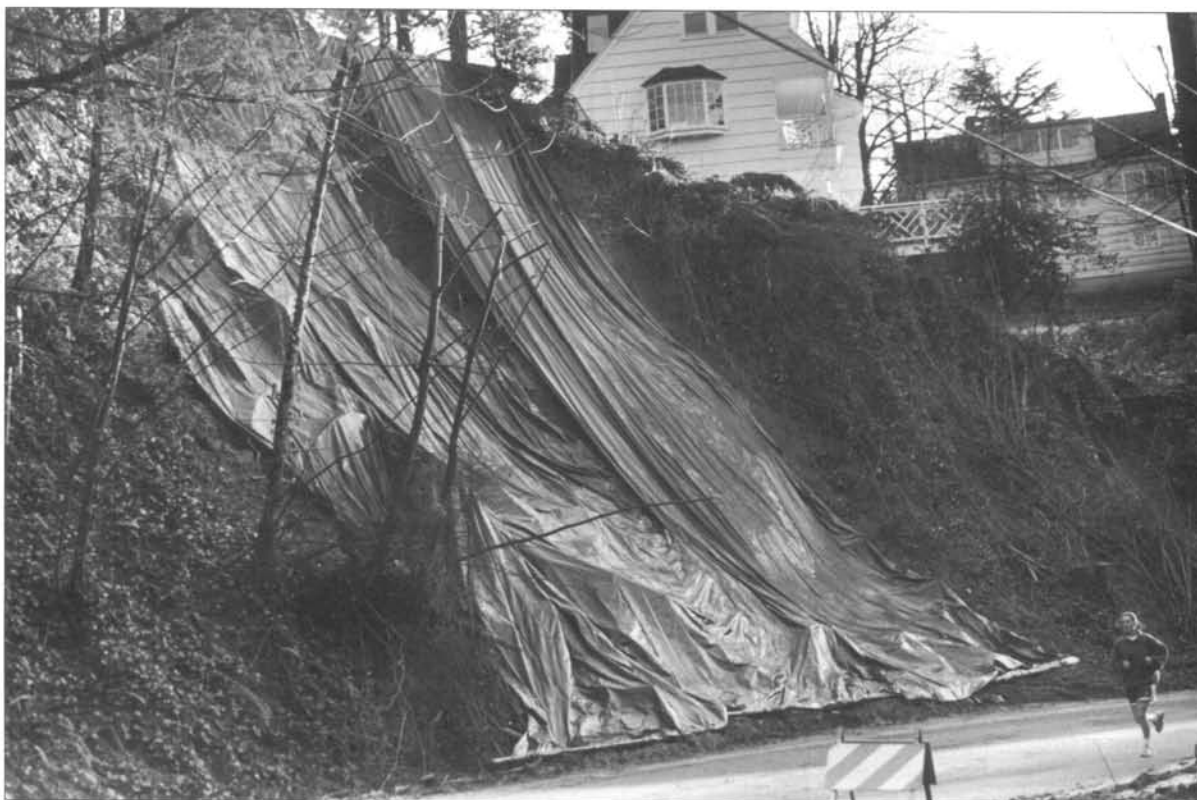
Slide on 2700 block of SW Fairmont. Plastic covers the slope to keep rainwater away from it.
