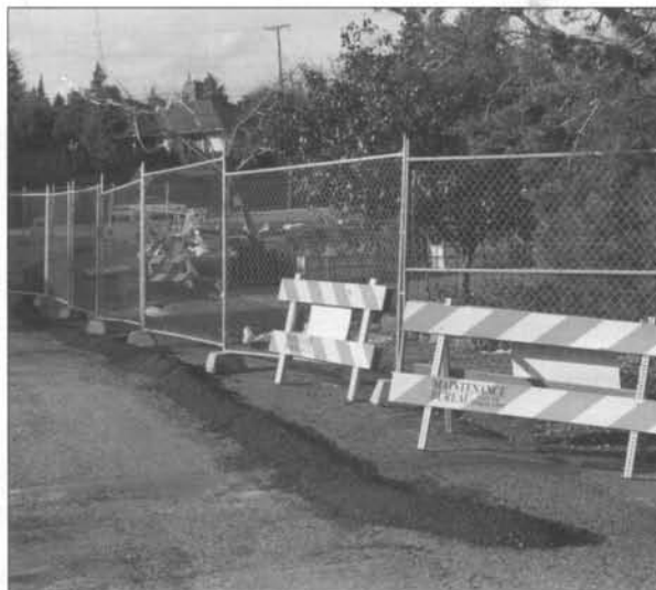
Asphalt berm placed on edge of SW Council Crest Drive to keep water from running over edge of road and flowing onto landslide below the road.
