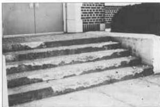
Figure 3. Damage to Molalla High School, Molalla, Oregon, from the Scotts Mills earthquake of 1993. Bricks from the unreinforced masonry gable over the doorway fell to the steps and sidewalk (left photo) during the earthquake, illustrating the need for seismic rehabilitation. The damage to the steps (right photo) that was revealed when the debris was removed can serve as a vivid reminder of an important rule for response during an earthquake: Do not run out of a building! Rather, "duck, cover, and hold!"
