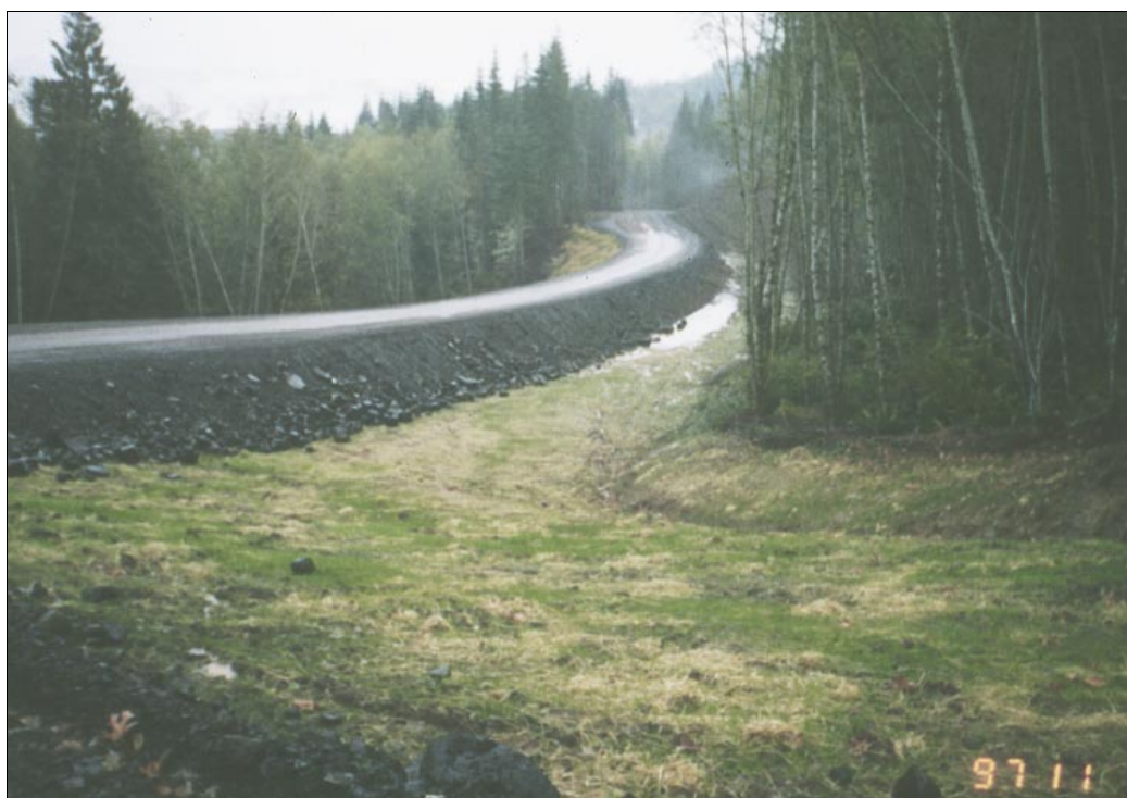
Rebuilt access road in quarry operation of Coos County Road Department near Myrtle Point, commended for control of erosion and storm water runoff.
