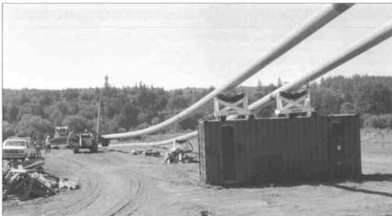
Above and on facing page: Installation of natural gas pipelines was part of the Northwest Natural development of the Calvin Creek gas storage project at Mist Gas field. While the pipes were being assembled, they were temporarily suspended above Highway 202 near Mist, Oregon, before they were permanently buried deep underground—and under the highway.
