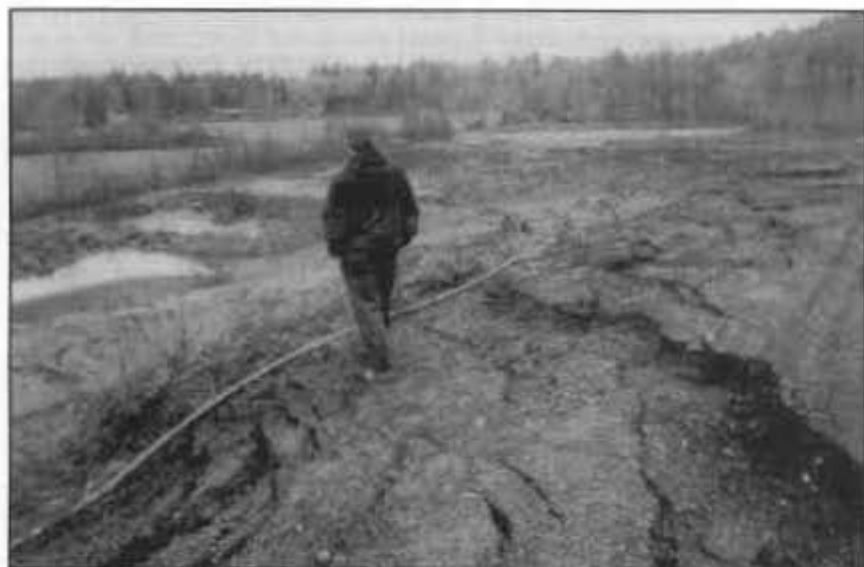
Figure 3. Slope failure at American Sand and Gravel site below processing area. Impacted wetlands located in background. Photo taken in 1993 by E. Frank Schnitzer.
