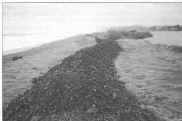
Figure 7. Erosion at Port Orford, north of The Heads, during the 1997–98 El Niño event. View is to the south from the location of Figure 6. The erosion is now threatening to break through the beach/dune barrier and wash into Garrison Lake, which is being prevented by the placement of a gravel ridge.
