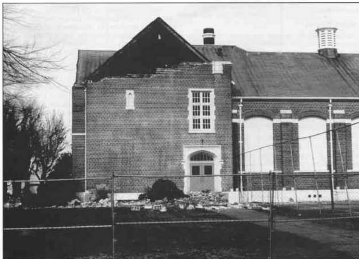
Figure 1. Earthquake damage at Molalla High School from the Scotts Mills ("Spring Break") earthquake, March 25, 1993.
