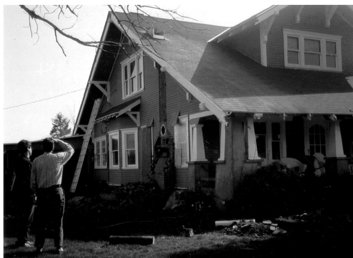
Chimneys, usually built of unreinforced masonry, show the most common type of damage caused by the 1993 Scotts Mills earthquake. Photos show house near Molalla on left and roof of authors' home near Scotts Mills (right). Photos courtesy of Doug Eaton.
