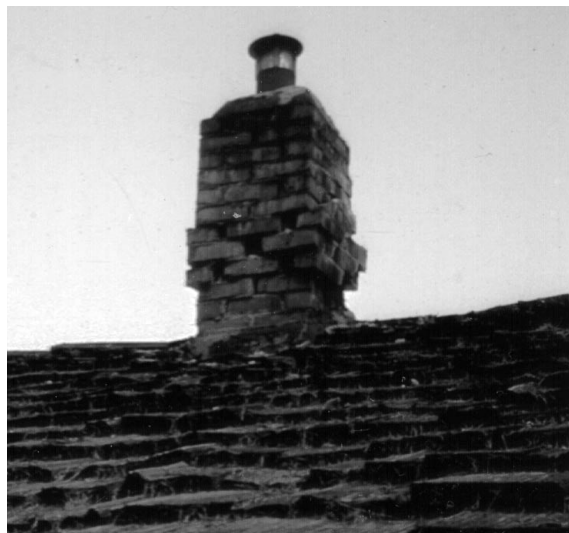
Chimneys, usually built of unreinforced masonry, show the most common type of damage caused by the 1993 Scotts Mills earthquake. Photos show house near Molalla on left and roof of authors' home near Scotts Mills (right). Photos courtesy of Doug Eaton.
