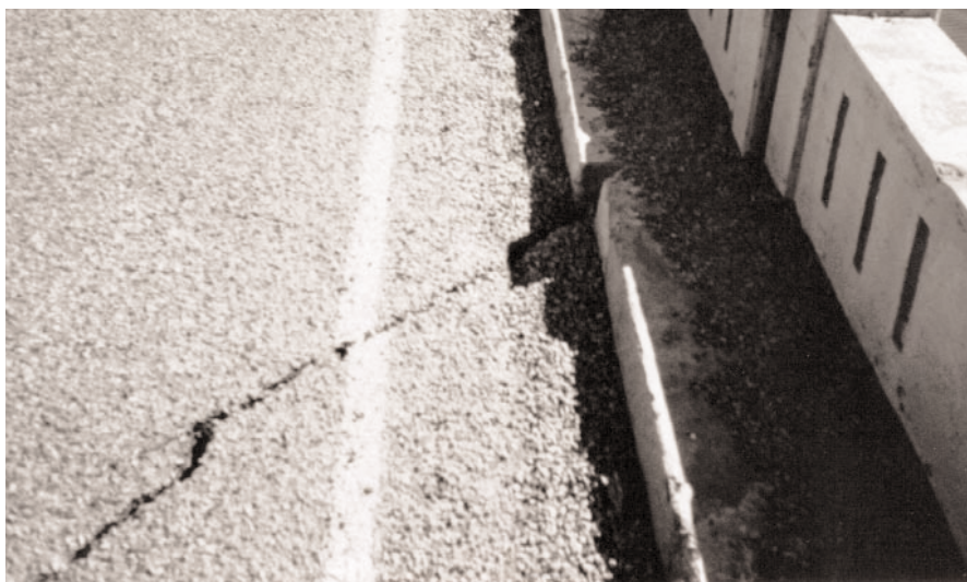
Two people died in the 1993 earthquakes in Klamath Falls. This bridge on Hwy 140 shows left lateral displacement across joints in the bridge deck, probably as a result of slumping and settling that caused the bridge deck to rotate.
