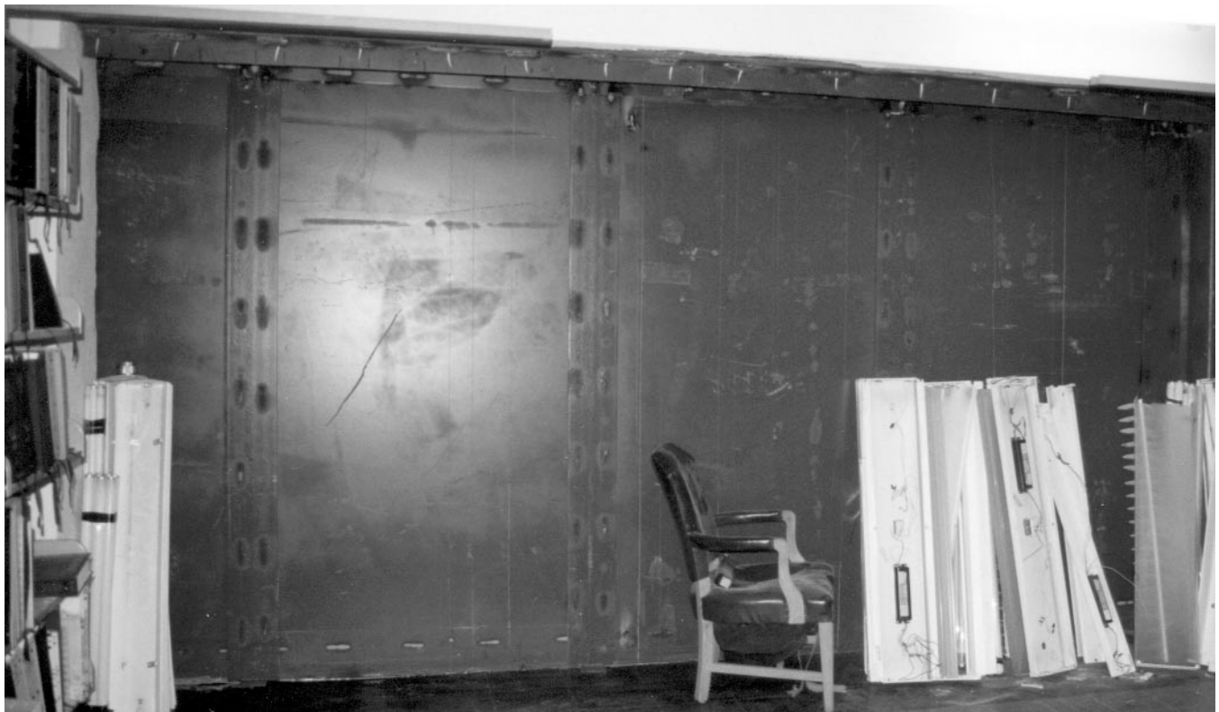
Example of steel-plate shear wall in basement of Oregon State Library during construction.
