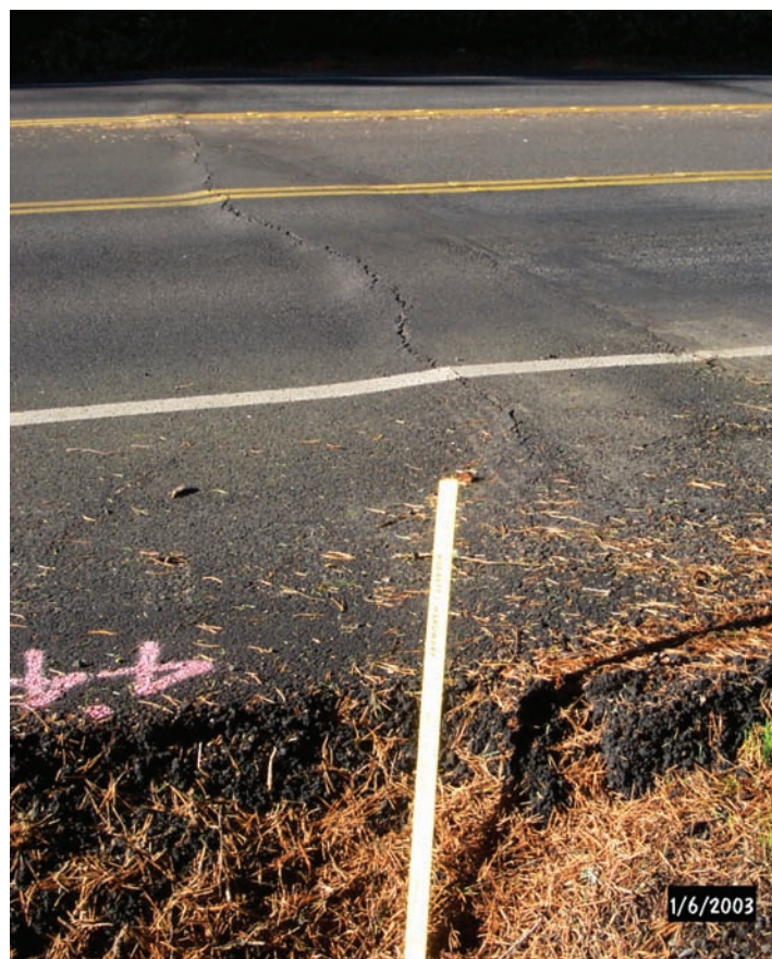
Figure 25. Damage to the north slide margin on Highway 101 from the same movement as in Figure 24. Note that vertical offset is only 1-2 cm.
