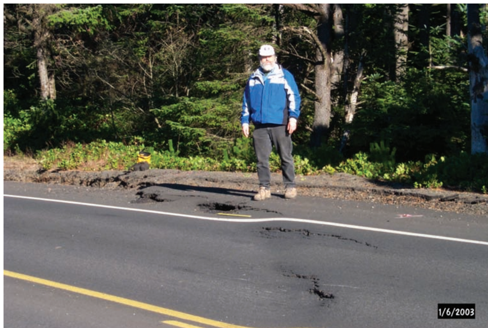
Figure 24. Damage to Highway 101 on the south margin of the Johnson Creek landslide immediately after a slide movement in January 2003. Maximum vertical offset is 17.8 cm down to the northwest; fissures are as wide as 5 cm. This part of the slide is south of the resurvey lines and confirms the general trend of increasing offset to the south. Roger Hart is in the background.
