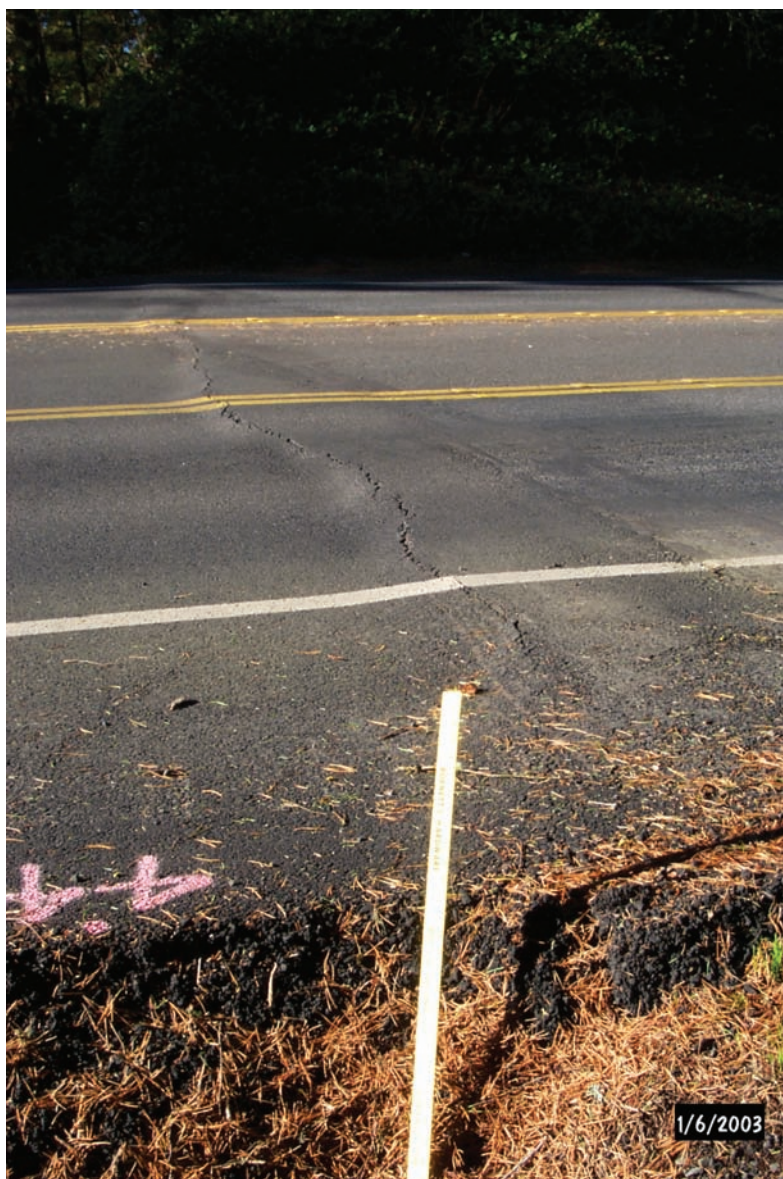
Figure E10. Damage to the north slide margin from the same movement as in Figure E9. Note that offset is only 1-2 cm vertical.
